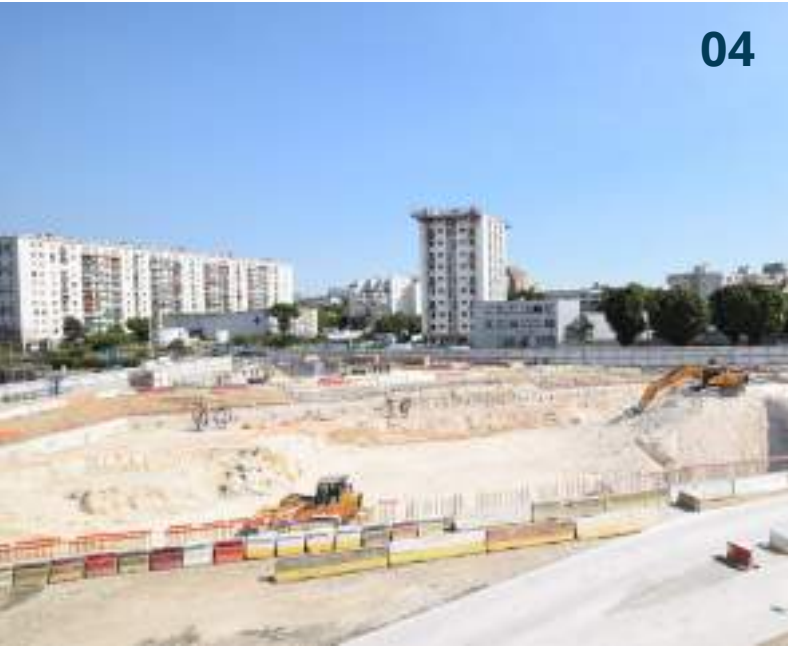
04 Grand Paris Express – Bagneux M4-15 Paris, France, 2016 Client: Franki Foundations
