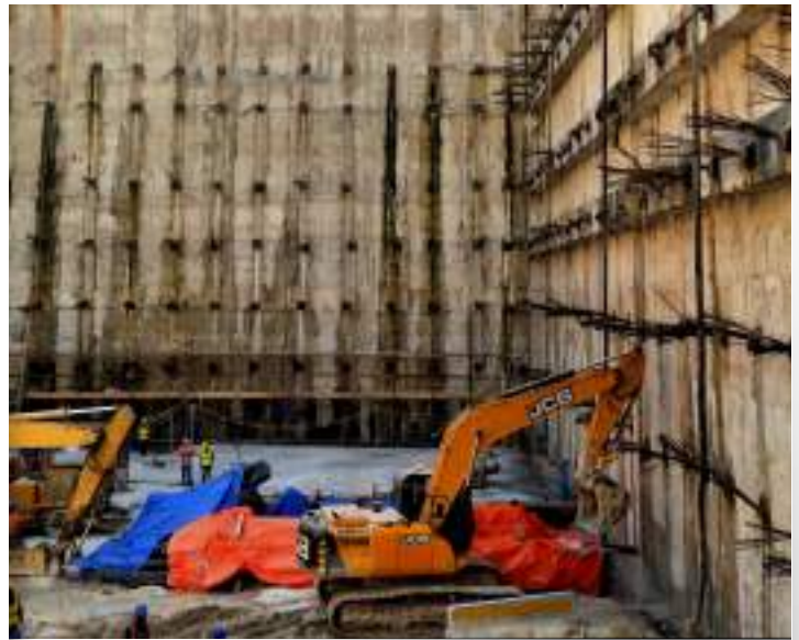
Soil retention & stabilization
